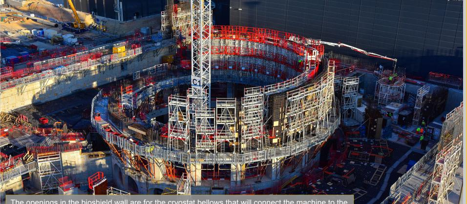
The openings in the bioshield wall are for the cryostat bellows that will connect the machine to the port cells designed to give access to systems such as remote handling, heating and diagnostics.
