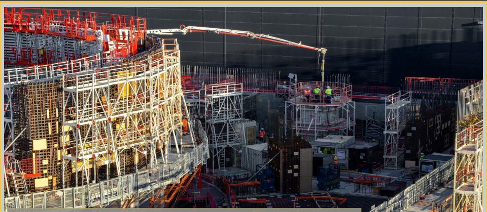
Eighteen massive columns will provide structural support to the Tokamak Complex. Here at the L2 level of the Tokamak Building, concrete is being poured into one of these "mega columns."
