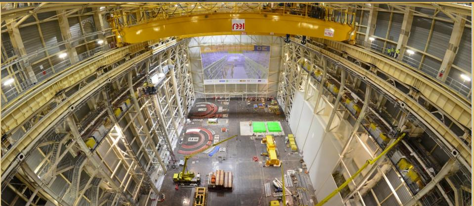
Before being integrated in the machine, the components will be prepared and pre-assembled in this 6,000 m2, 60-metre high building. The Assembly Hall is equipped with a double overhead travelling crane with a total lifting capacity of 1,500 tons.
