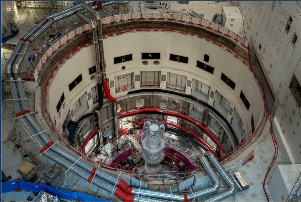
20 August 2021 – Central column (an in-pit assembly tool)
