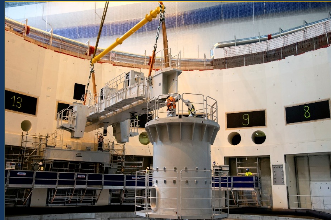
7-8 September 2021 – Test positioning of first radial beam (9 supports for the 9 sector modules – each 1000+ tonnes)
