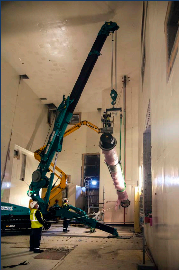
▲ Cryoline installation
