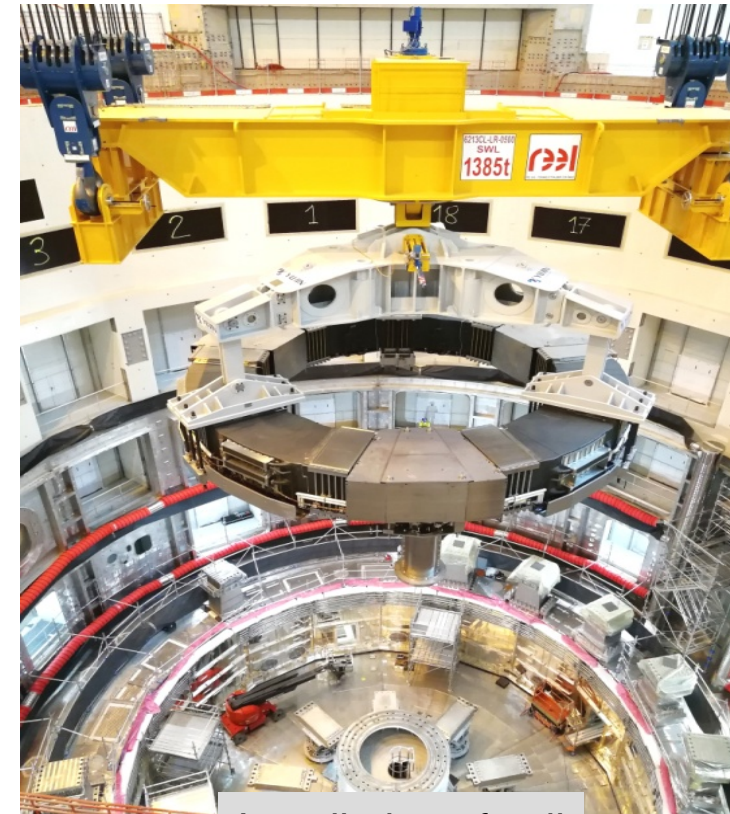
Installation of coil
