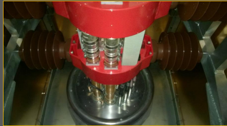
SPIDER TL connected to vacuum vessel electrical bushing.
