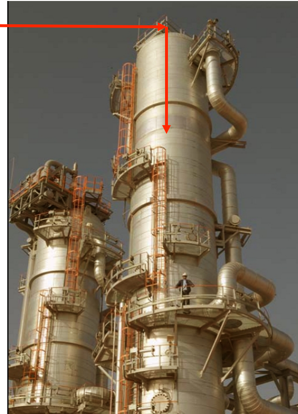
Amine contactor towers
